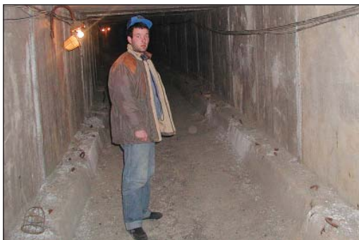
Where the sun doesn’t shine. In winter, underground tunnels are often the only way for technician Tigran Yepiscoposian and others to move between buildings.
