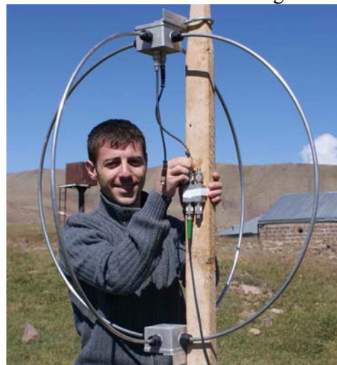
David Pokhsroryan Installing Antenna
